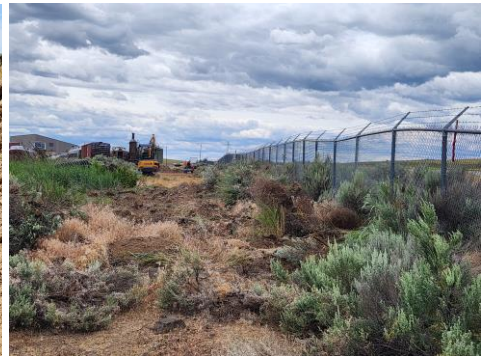
Tail track alignment, center line 15' from fence.
