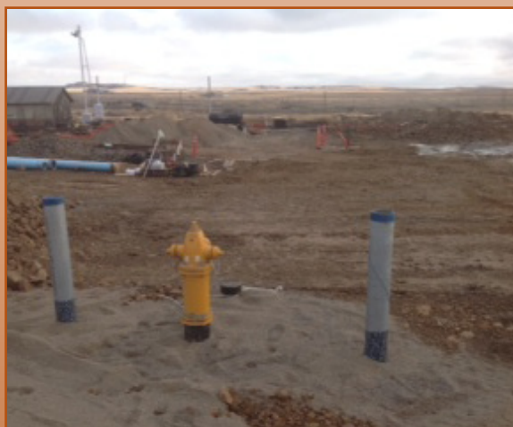
The fire system is backfilled and ready for the tanker car
