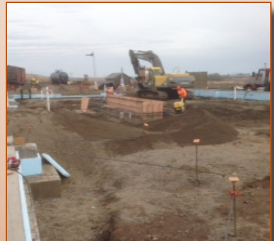
MJM Grand grading and compacting subgrade
