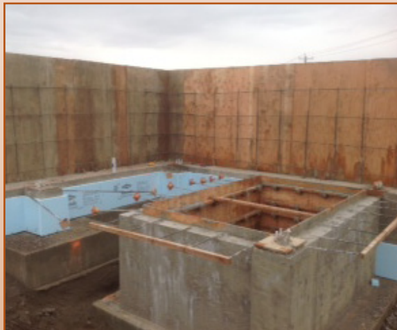
Elevator pit ready for waterproofing
