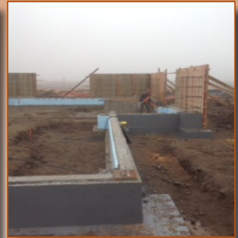
Stem walls are dampproofed, insulated and ready for backfill
